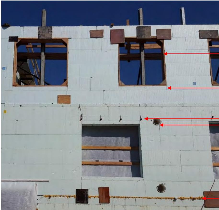
Integral cast insulated jamb are cleanest tightest detail
