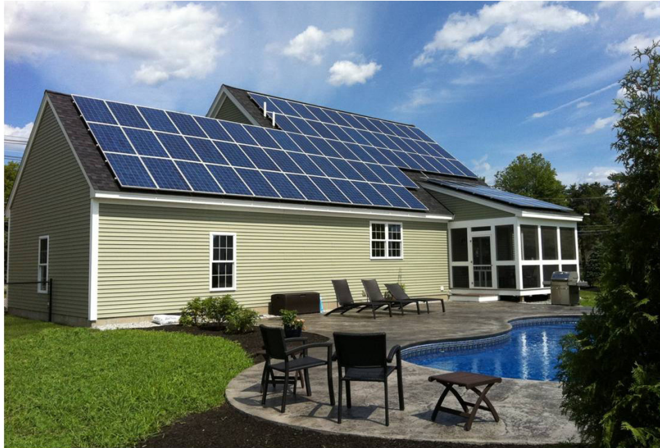
Cooler than a pool: This backyard PV system was estimated to produce enough extra power annually to run a Chevy Volt 30,000 miles.
