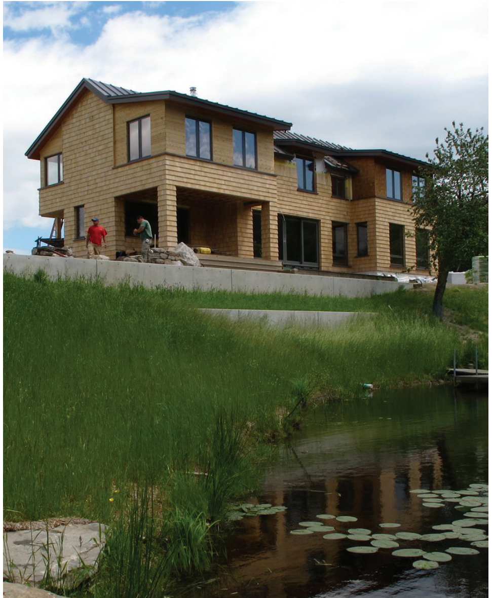
The owners of this Falmouth, ME, home got to net zero while preserving the building's original post and beam construction. See “before” on page 21.
