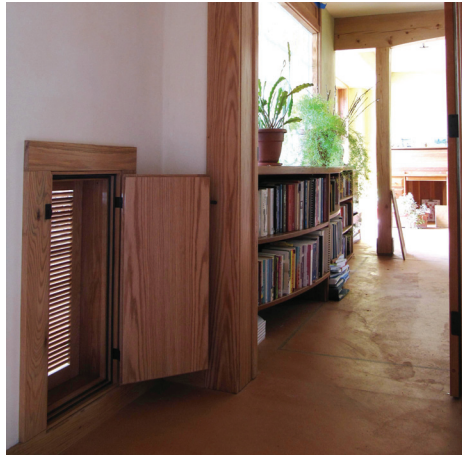
Louvers between rooms aid passive air circulation.
