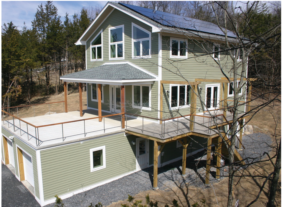
The Shepler residence is the first of 25 planned for Green Acres, a zero net energy community in New Paltz, NY. The home's 10 kW PV system provides enough power for both household needs and a future plug-in electric vehicle. Triple-glazed, krypton-filled windows are placed for solar gain in winter.
