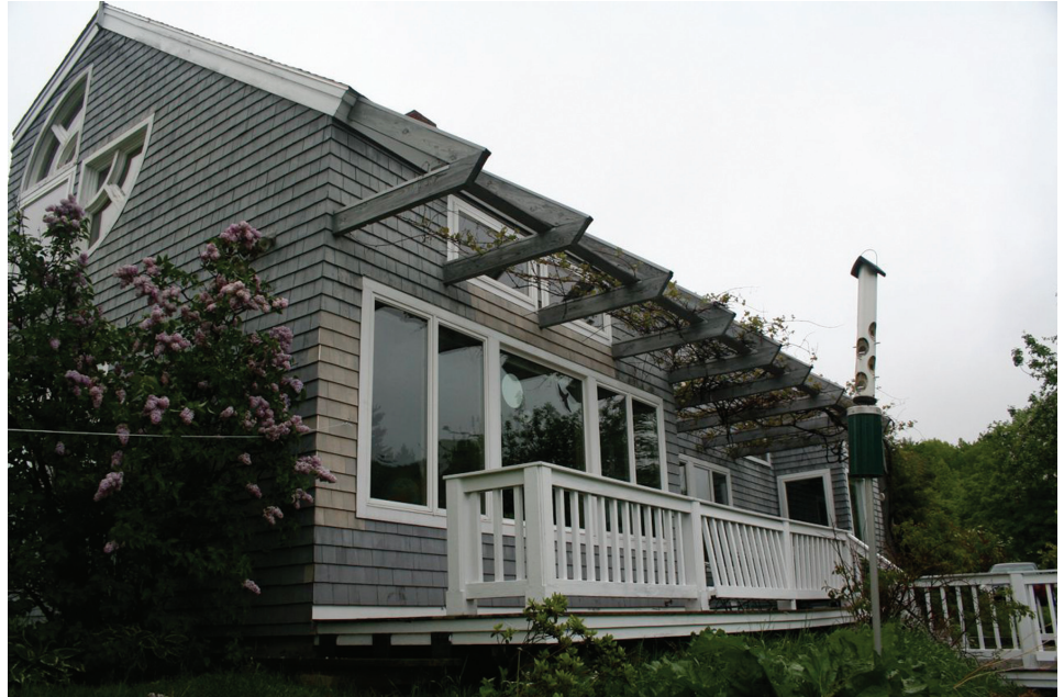
The original home, designed as a passive solar house in 1975, built up heat on sunny winter days only to release it quickly due to poor insulation and air sealing.
