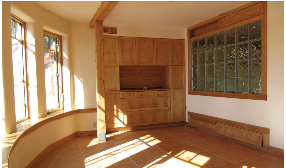
The glass wall is filled with water in a novel attempt to add thermal mass.
