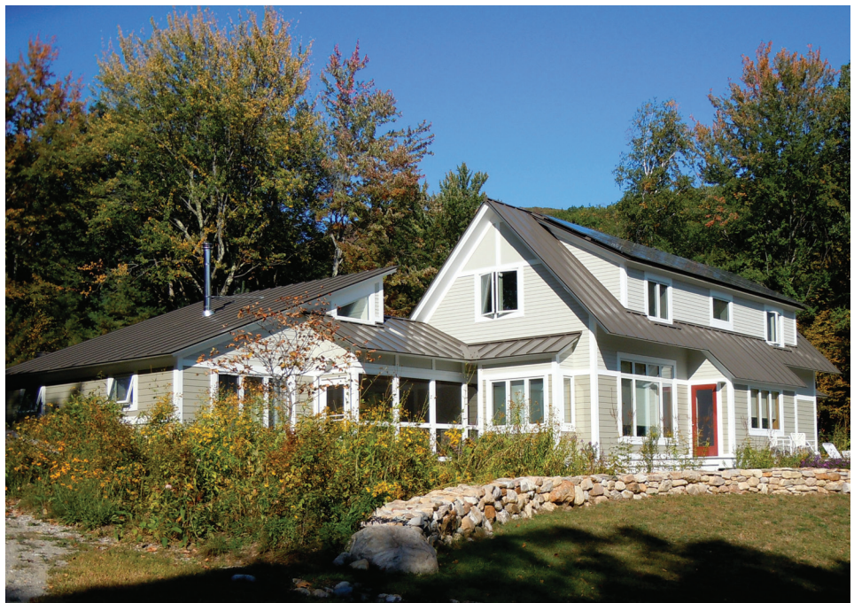
The Moomaw house, west elevation.
