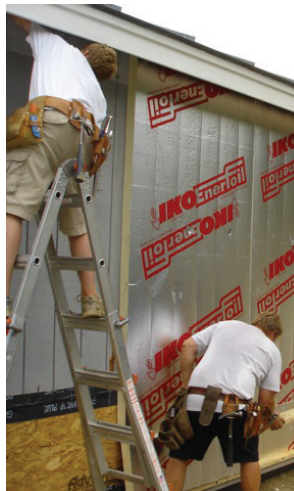
The insulation was radically upgraded.
