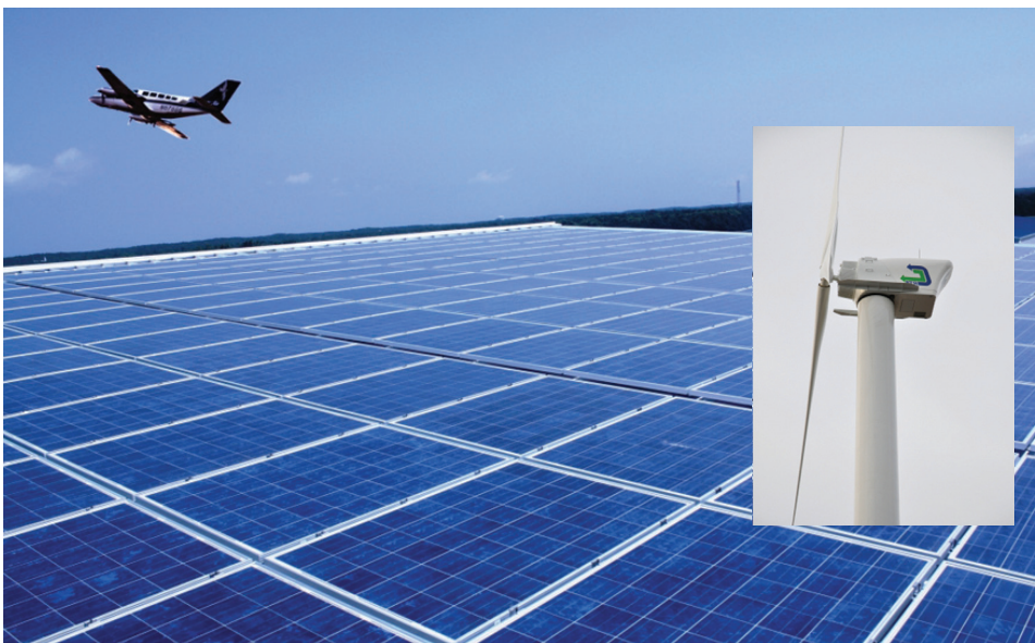
A Cape Air Plane soars over Cape Air's 258kW rooftop PV installation. Inset is the newly installed Northwind 100 turbine at the Cape Cod Regional Transit Authority.
