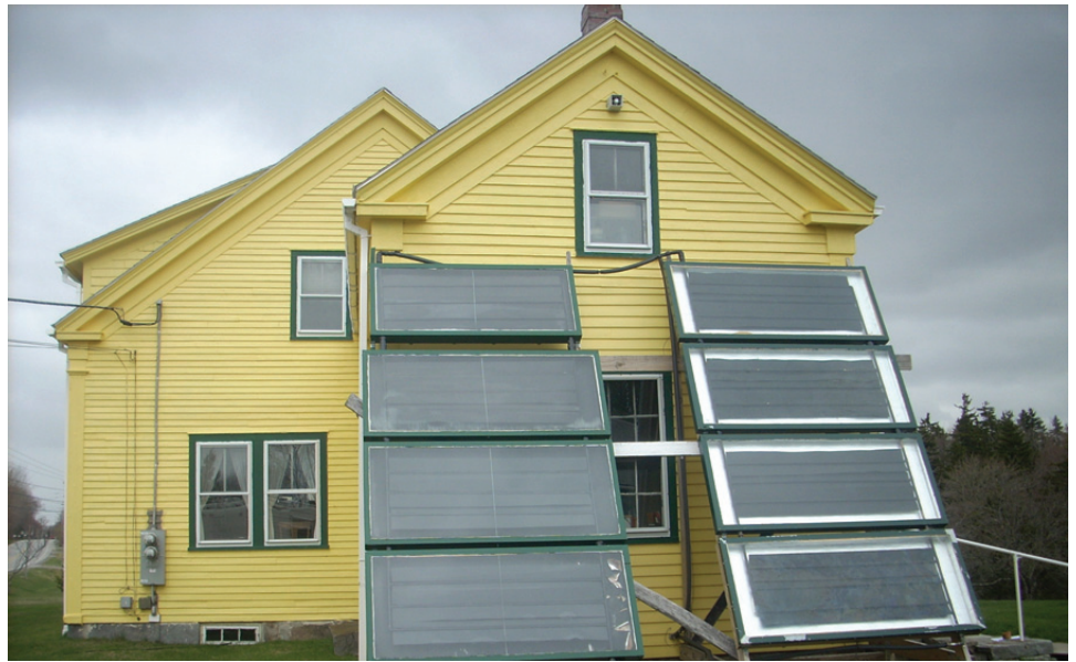
Assembly of this St. George, ME, farmhouse's hot water system started at a MeSEA workshop. It incorporates eight solar thermal collectors handmade from recycled glass and all local materials.
