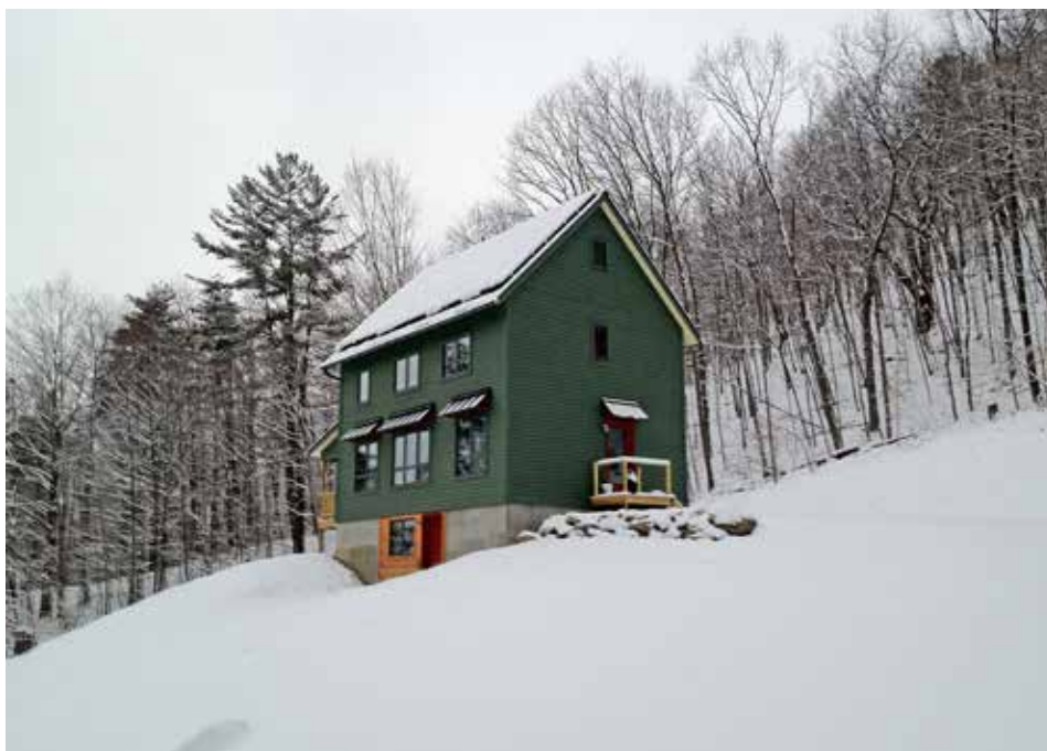
Upstate New York winters are no problem for the Burk House. The home/farmstead won on the strength of its comprehensive sustainable design, simple elegance, and educational component.
