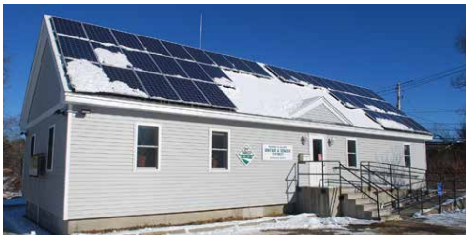
Post-retrofit, this Plymouth, New Hampshire, town office building consumes two-thirds less energy. It makes up the rest and then some with a 9 kW PV array.
