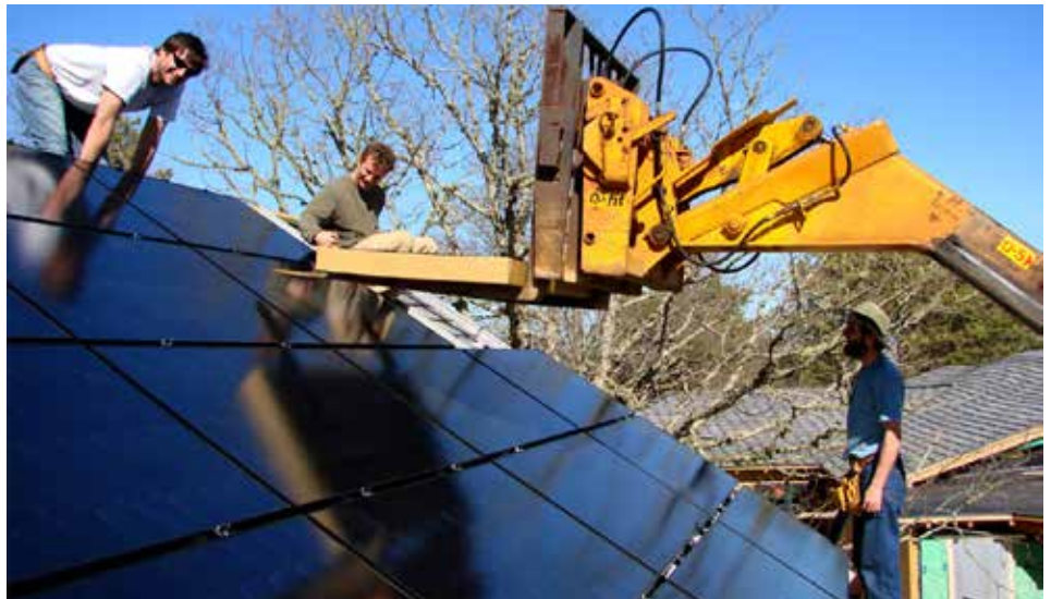
Last but not least is a renewable energy system. As prices fall, less-than-perfect apertures that have shading or don't face close to south become worth considering.
