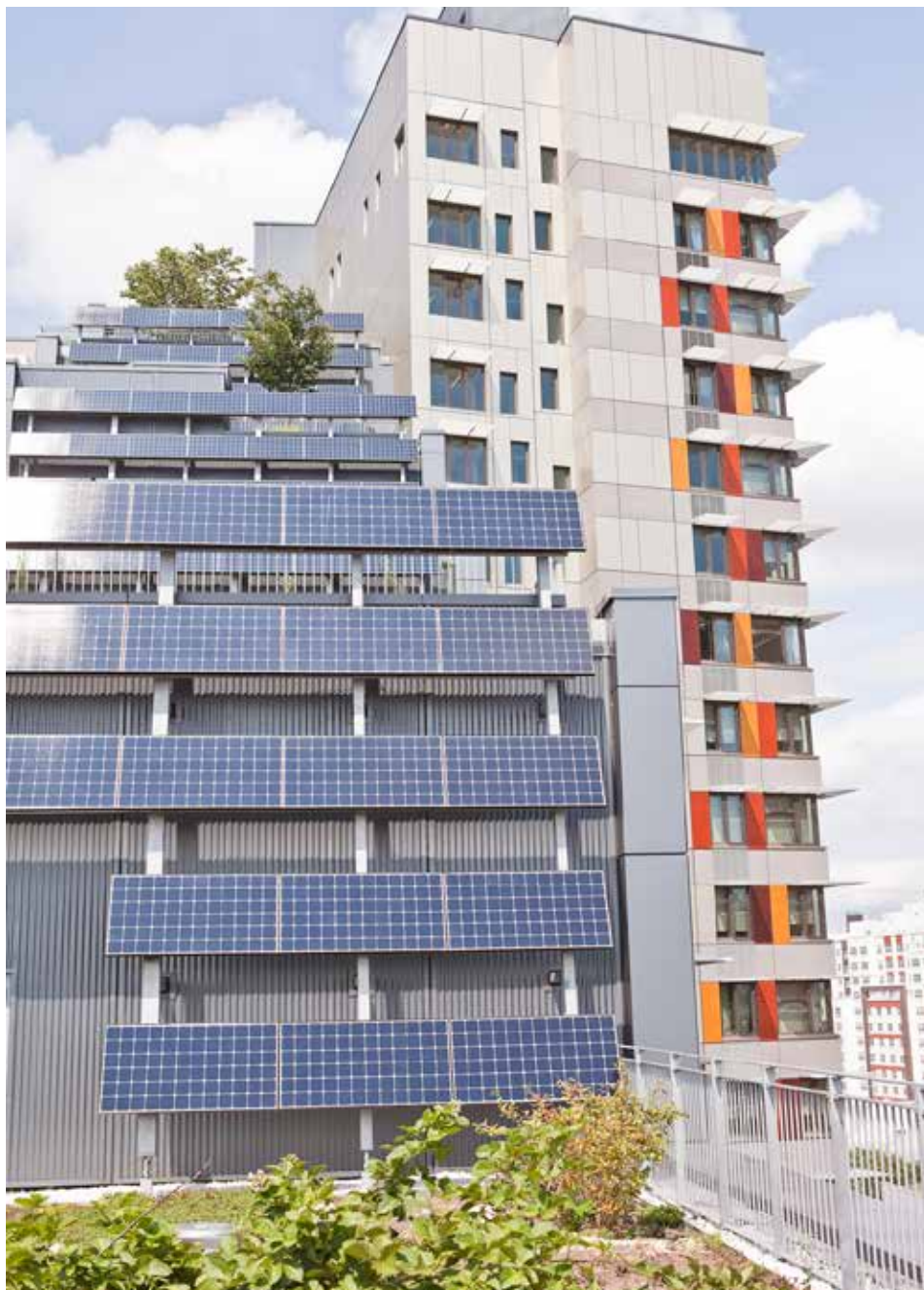
Solar in the city: Via Verde, a 222-unit affordable housing project in the Bronx, enjoys a 66-kw building-integrated solar electric system. The urban infill project also includes a green roof, community vegetable gardens, rainwater harvesting, and more. See viaverdenyc.com .
