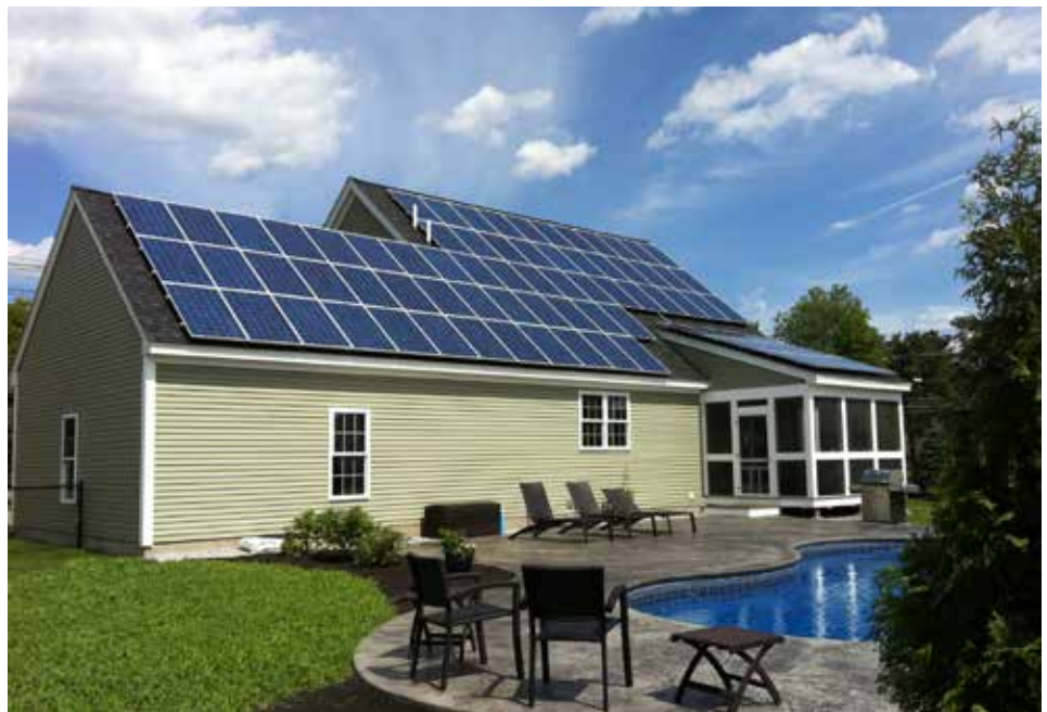
In each of the last two years, Transformations Inc.'s Nakuset Way has generated excess energy averaging more than 9,000 kWhs.
