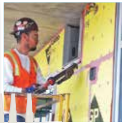
Joint & Seam Filler fill coat and seam treatment
