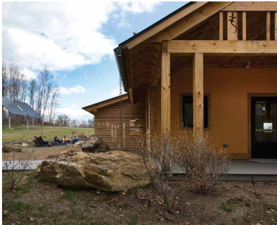
With the building site hard against a protected wetland tree line to the west, the project team pole-mounted two 4.8 kW Sunpower arrays, seen here beyond the entry porch.
