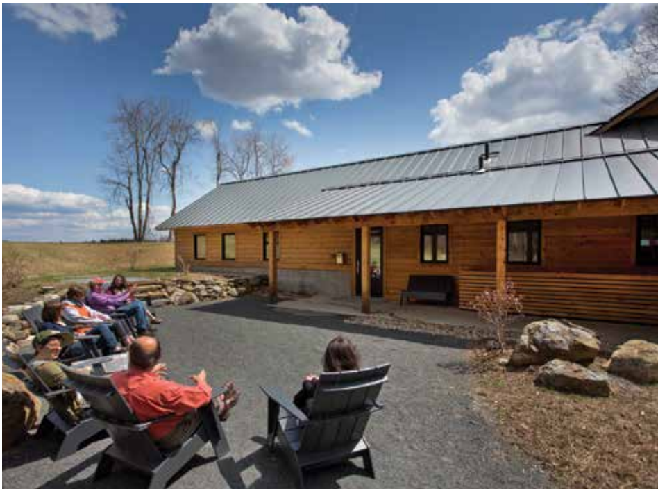
Salvaged cypress siding and locally and regionally harvested FSC lumber and glulams met the requirements of the LBC’s “Materials” petal.
