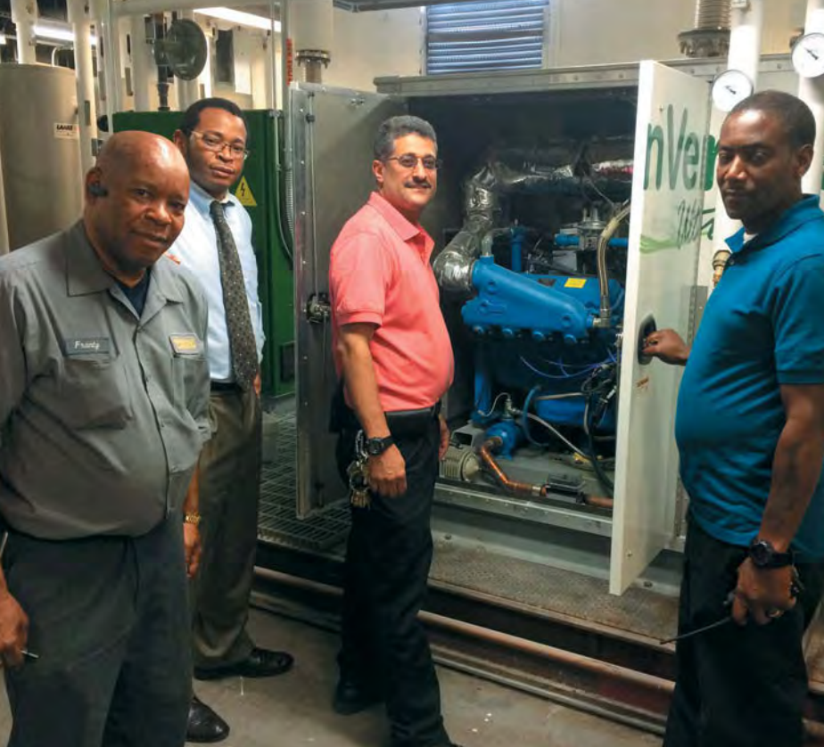
A TEAM INSPECTS HVAC EQUIPMENT AT ROOSEVELT LANDINGS ON JUNE 20, 2014.
