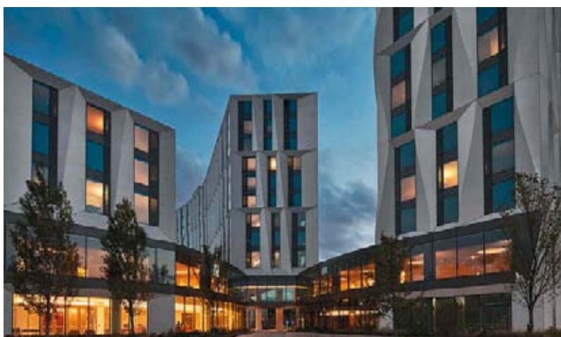
THE UNIVERSITY OF CHICAGO CHOSE A SITE GOAL OF 55 KBTU/FT 2 -YR FOR THE 390,000-SQUARE-FOOT RESIDENCE HALL AND INCLUDED THAT TARGET IN THE RFQ. PHOTO CREDIT: THE UNIVERSITY OF CHICAGO.
