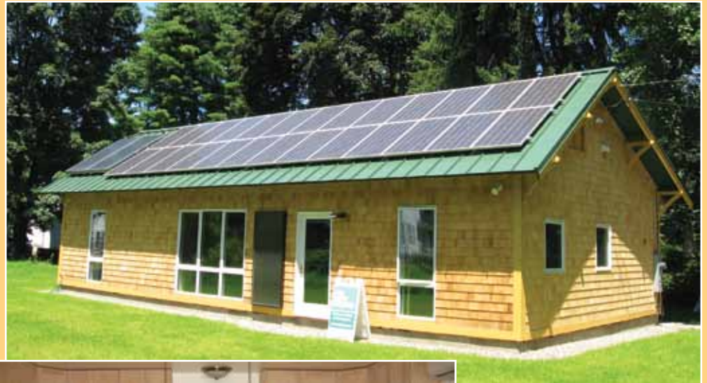
Assorted pictures from Tina Clarke and Doug Stephens' Montague Urban Homestead, Turners Falls, MA. Clockwise from top: South-facing exterior with grid-tied 4.94Kw PV system and two 4' x 8' flat plate collectors, entry way with cork floor, 12" double-stud walls with dense-packed cellulose insulation, and kitchen with cork floor and Energy Star® appliances.
