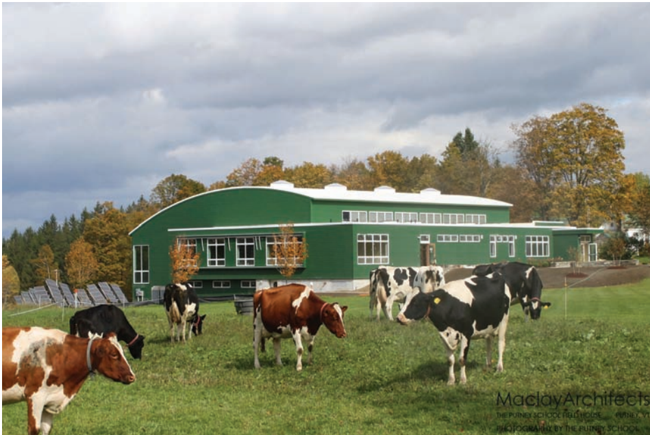
The Putney School Field House, at 17,000 square feet, now has three years of documented zero net energy use under its belt.
