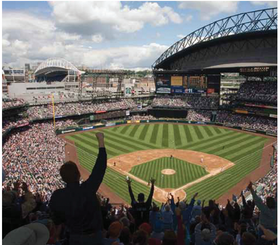
The Seattle Mariners' Safeco Field. Energy-saving upgrades to lighting and more have saved the team over $1.75 million since 2006. A 32.76-kW double-panel solar array (both sides absorb energy) is expected to generate 40,000 kWh annually.
