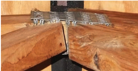
Deteriorated structural elements are surprisingly common. Among the potential problems are poorly selected wood members (e.g. knots), plate installation errors, and trusses with poor connection details and inadequate bracing. The roof at right collapsed due to a failed end connection.
