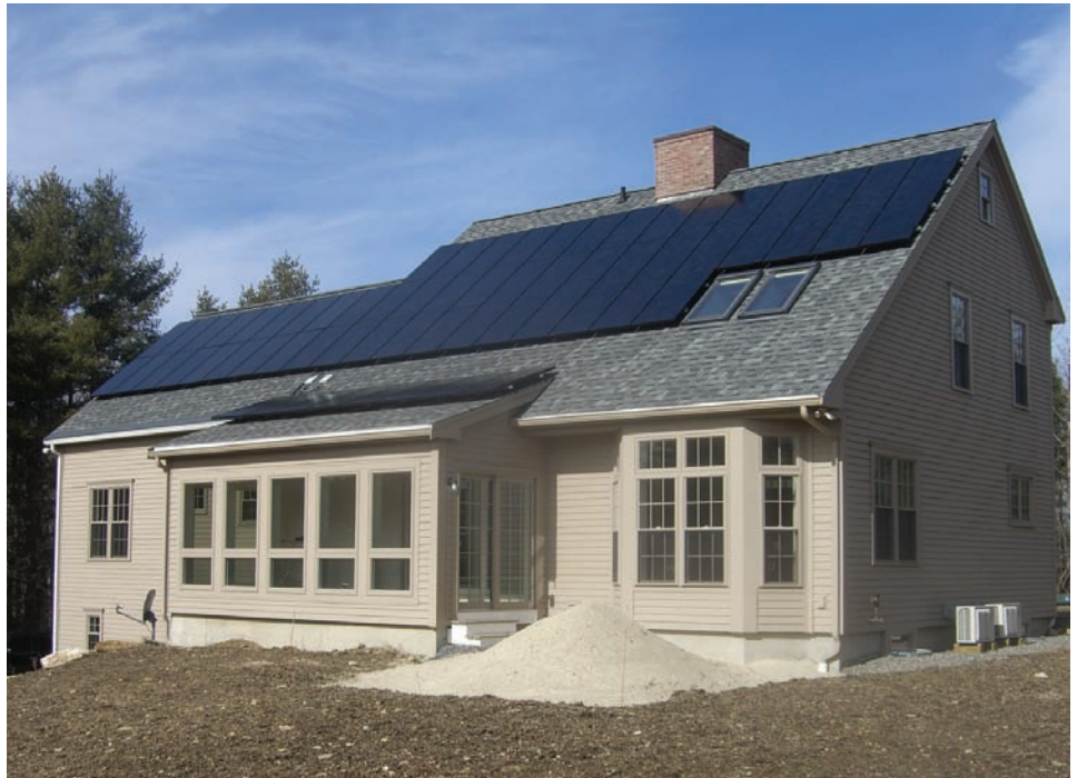
Built by Transformations Inc., superinsulated Nakuset Way consumed just 5,331 kWh of electricity during the year of monitoring. The PV's excess could power a car for 32,000 miles.
