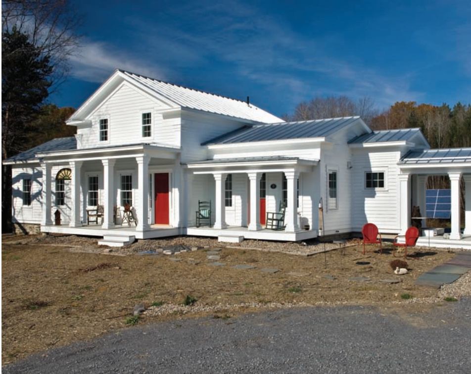
The Coons residence, an 1830s Greek Revival, had been vacant for 10 years before being both restored to its former stature and brought into the 21st century. The PV system—sited in the backyard to preserve the character of the house—powers the house and two electric cars.
