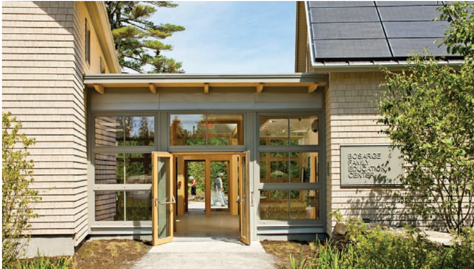
The building offers a welcoming gateway to the center’s classroom space and the botanical gardens beyond, while achieving the zero net energy and LEED Platinum goals set by the major donors.
