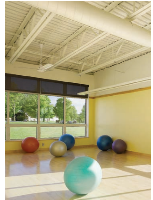
Triple-glazed, low U-factor skylights and windows allow natural light into the gym.
