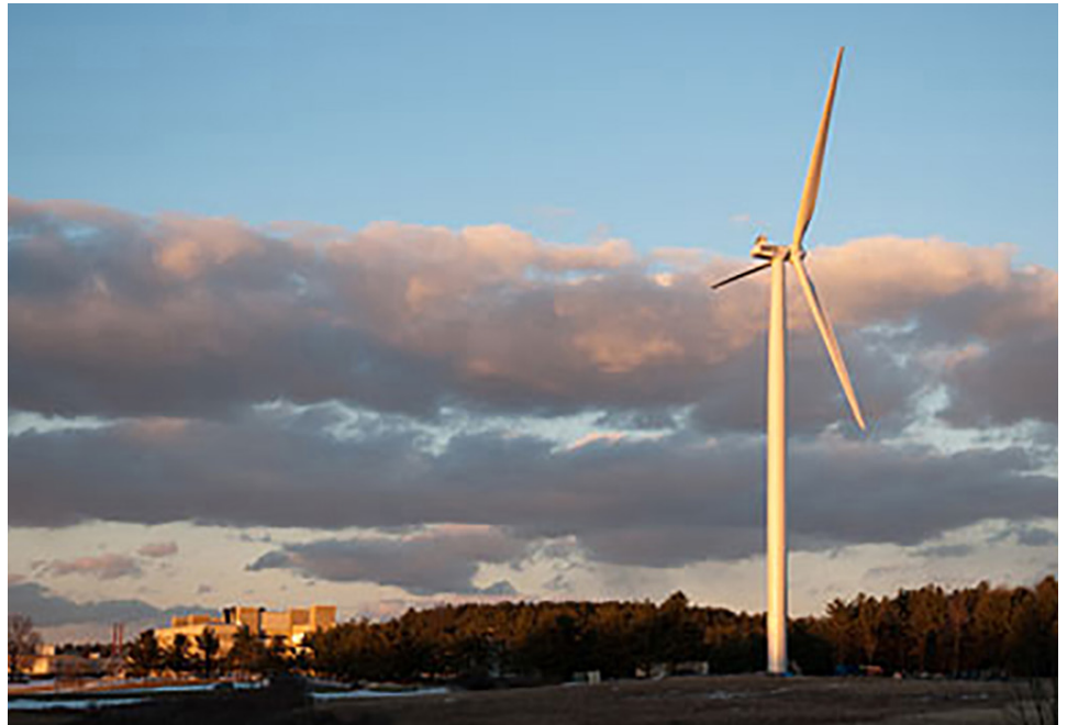
One of two 1.6 MW wind turbines installed at Mount Wachusett Community College in Gardner, Massachusetts. These supply all of the college's annual electricity requirements along with excess, which is sold back to the grid.
