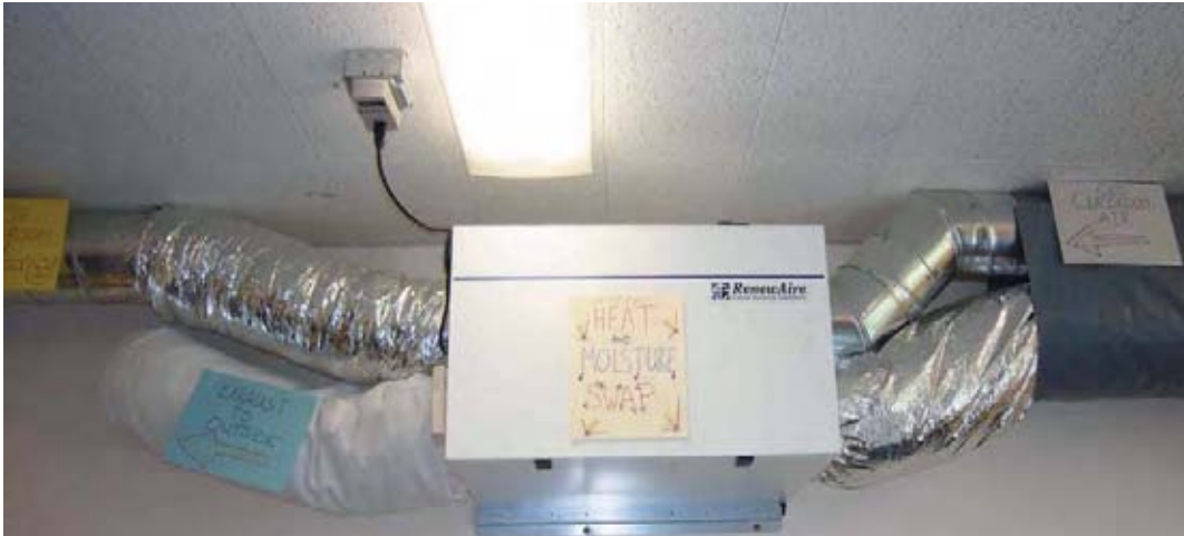
THE RENEWAIRE EV200 ERV UNIT RECOVERS BOTH SENSIBLE HEAT AND MOISTURE FROM THE EXHAUST AIR AND TRANSFERS THEM TO THE FRESH AIR. PHOTO CREDIT: MARC ROSENBAUM.
