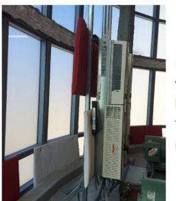
Foam panel vibration isolation inside the Radian penthouse.
