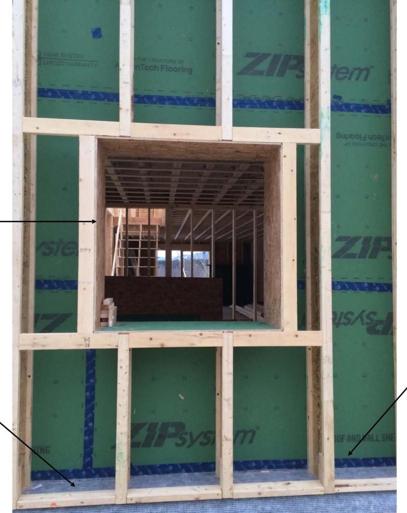
Subslab vapor barrier taped to zip first
