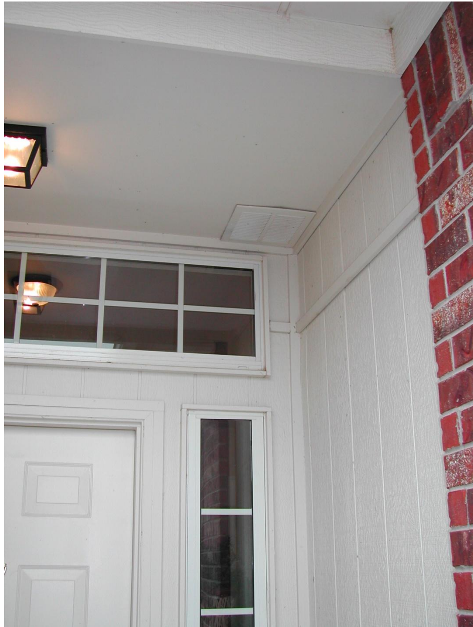
Outdoor air ducted to the return side of an air handler provides good distribution
