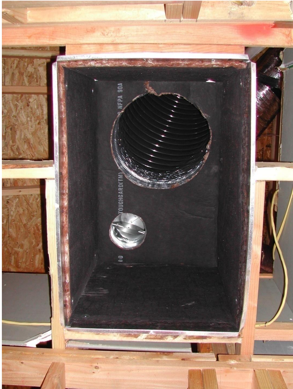
Outdoor air ducted to the return side of an air handler provides good distribution
