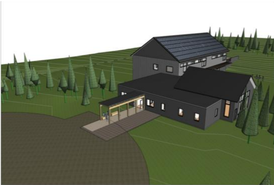
1A. General aerial view
