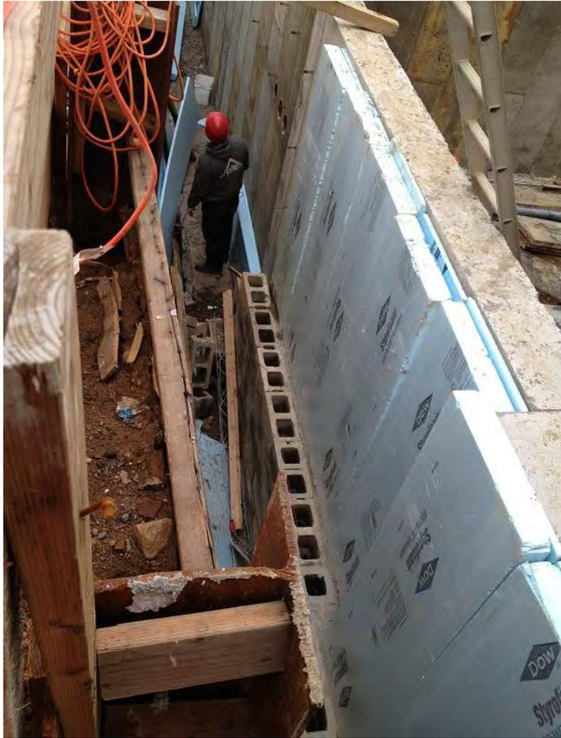
Installation of 5" insulation and CMU block is in progress
