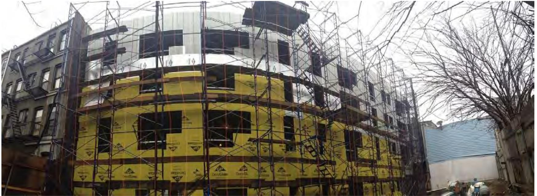
Back Facade – Pipe scaffold 100% up, Syntheon 100% complete, Densglass sheathing 60% complete
