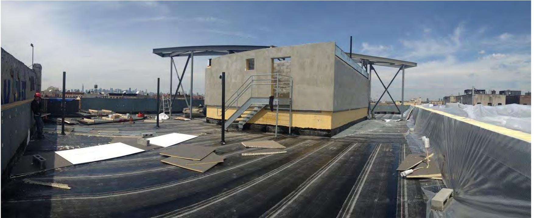
Roof – Bulkhead EIFS 60% complete, 1st ply of roof and crickets 80% complete
