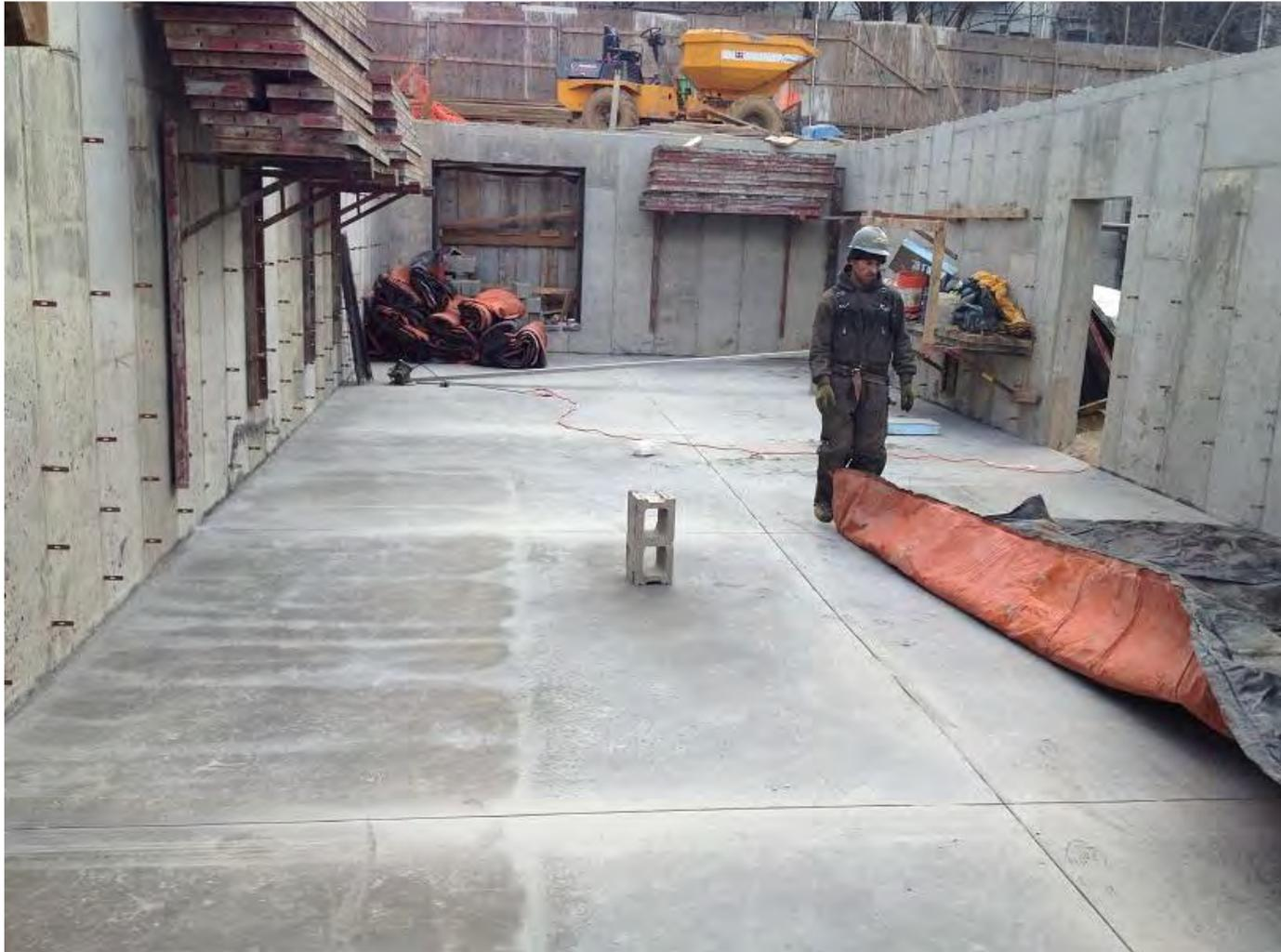
Community room slab completed. Heat retention blankets being laid.
