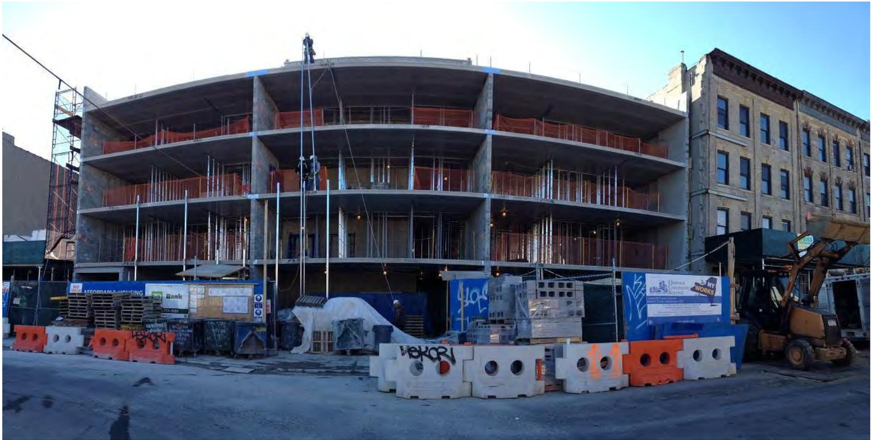
Front Facade – Pipe scaffold in place on left, Syntheon front facade studs install in progress
