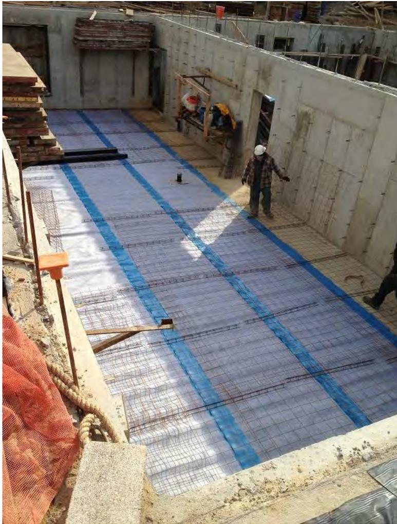
Vapor barrier, rebar mat for slab
