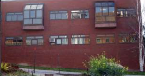
East elevation view
