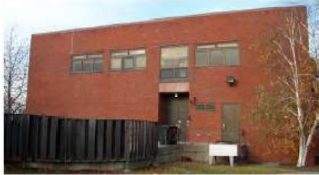
South East elevation view
