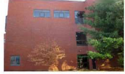
North elevation view
