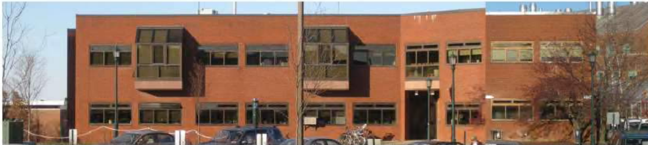
South Elevation View
