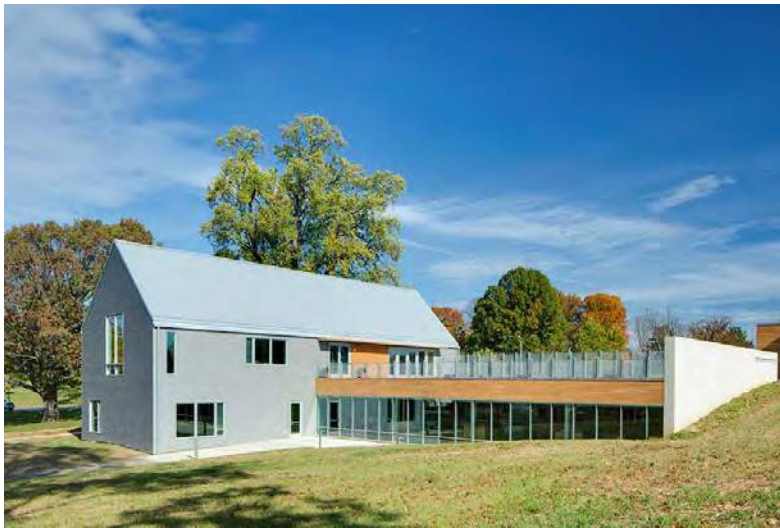
Headquarters building (10,000 SF)
