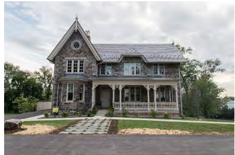
Superintendent's building (4,700 SF)
