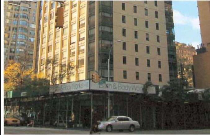
Tower East, New York, NY
