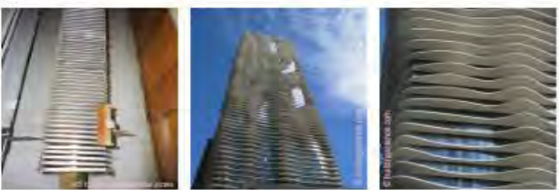
Photograph 1c (left): Extended Finned Surface - Aluminum; Photograph 1d (middle): Extended Finned Surface - Concrete; Photograph 1e (right): Aqua Tower Balcony's
