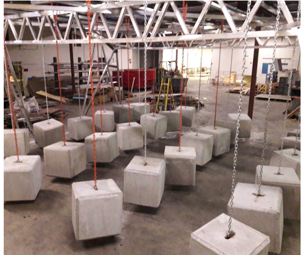
Maley Laser manufacturing facility Warwick, R.I., 2018
