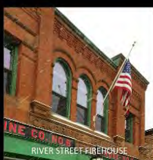
RIVER STREET FIREHOUSE
