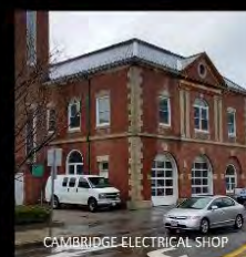
CAMBRIDGE ELECTRICAL SHOP
