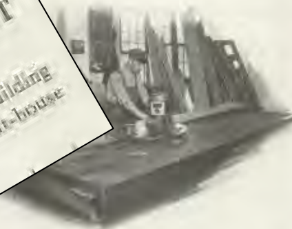
A Better-Built idea—routing (instead of cleating) stair-stringers for fine workmanship, and accurate fit.
