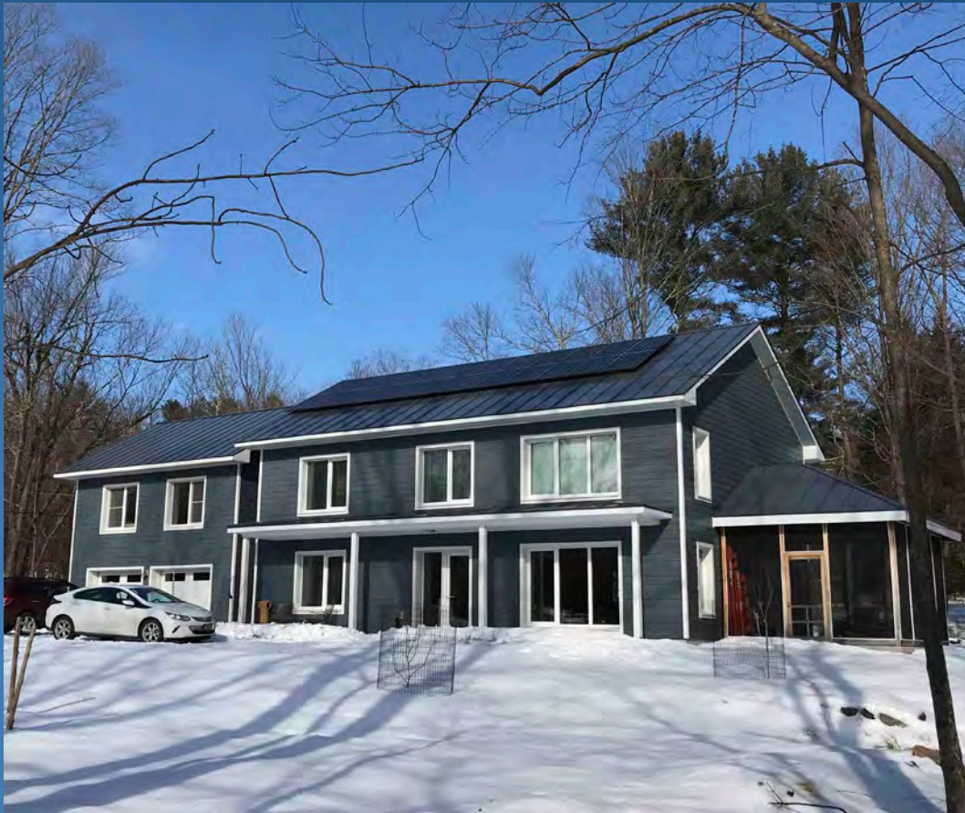
Passive House-certified Levy residence (built of AAC) in Woodstock, NY - photo: Alex Wilson
