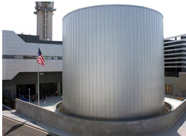
Thermal energy storage
