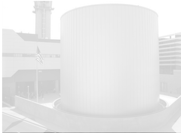
Thermal energy storage
