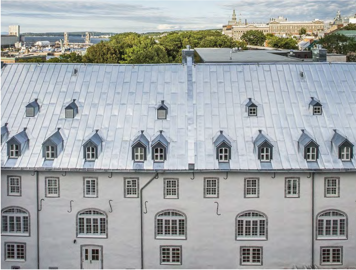
Wood windows and roof
