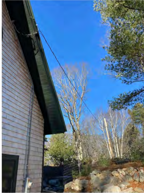
Photo of overhead span
