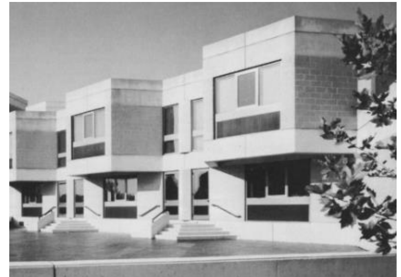
TMVL Existing Building Plan and Photos
