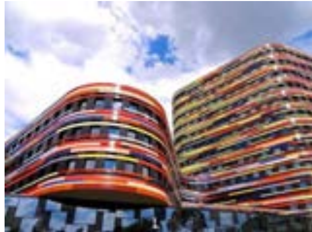
Ministry of Urban Development Sauerbruch Hutton Hamburg, Germany,
