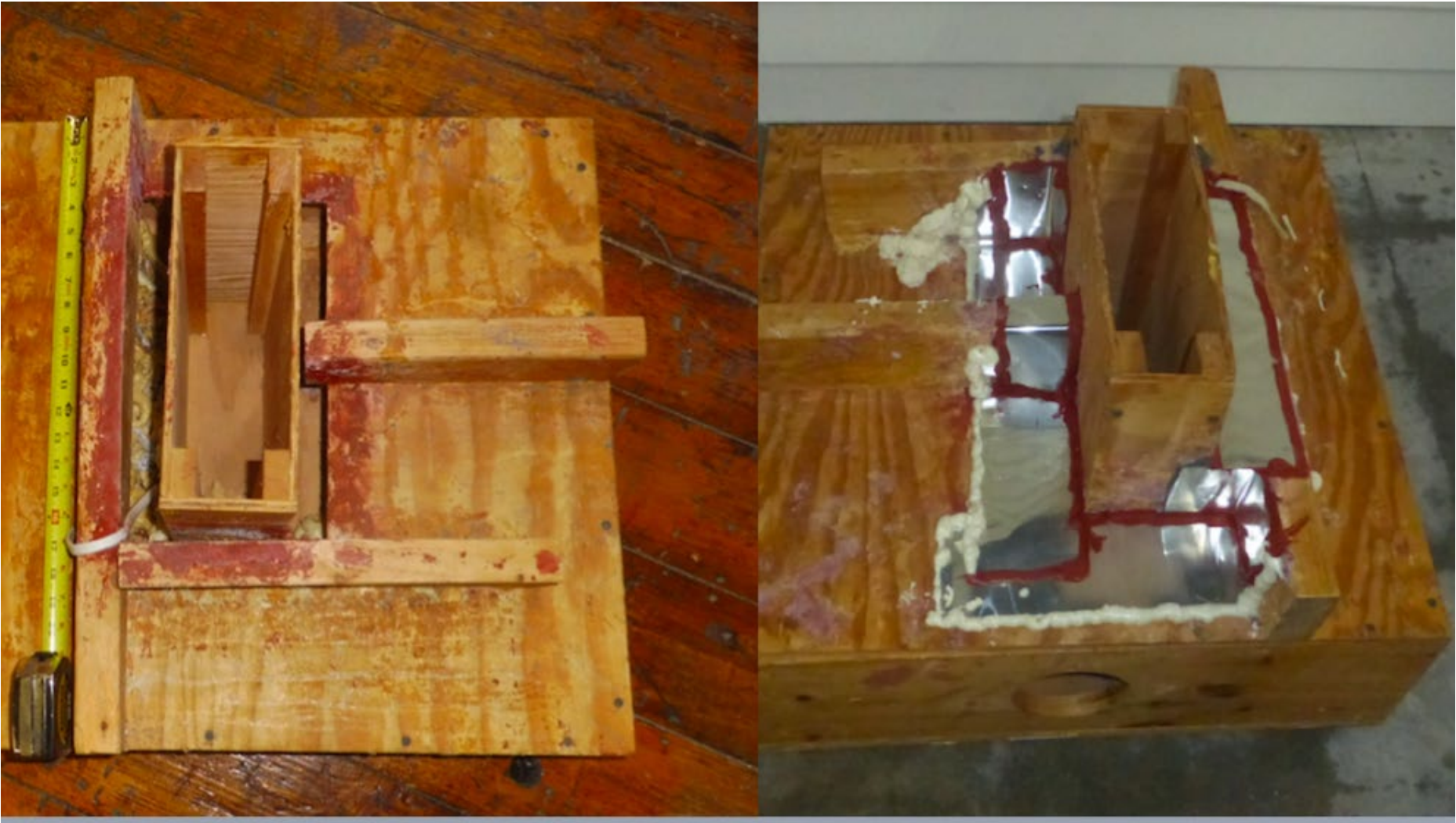
Attic Air Sealing Prop / Before & After
