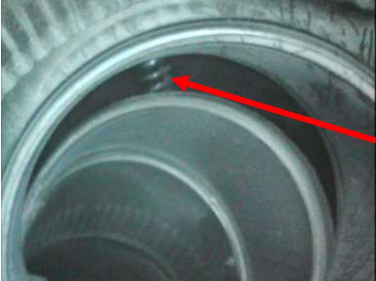
Duct Leakage
