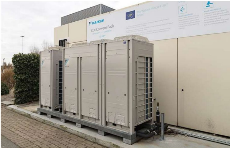
BELGIUM: Tests on an optimised CO2 version of Daikin's Conveni-Pack refrigeration system is said to have shown 21% lower life cycle emissions compared to traditional R410A.
