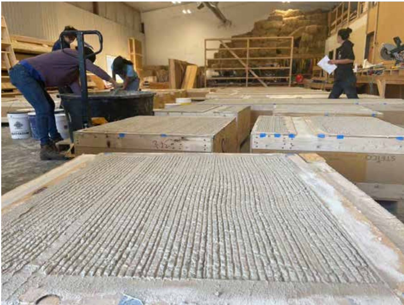
Local lime & clay plasters
