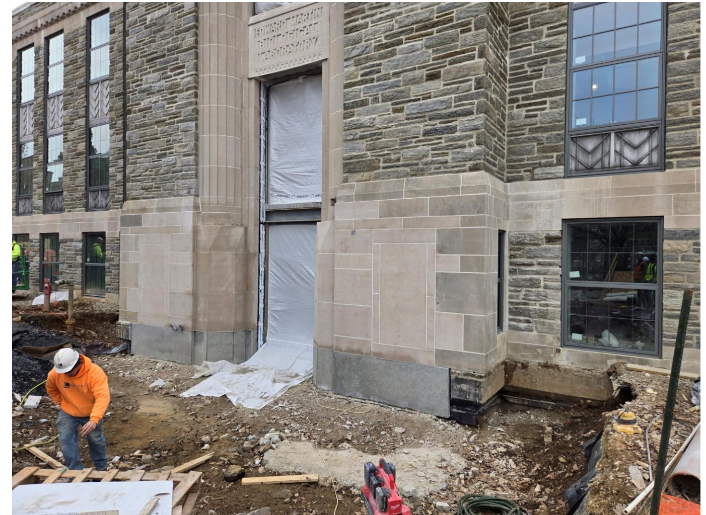
CONSTRUCTION PROGRESS (FEBRUARY '25)
