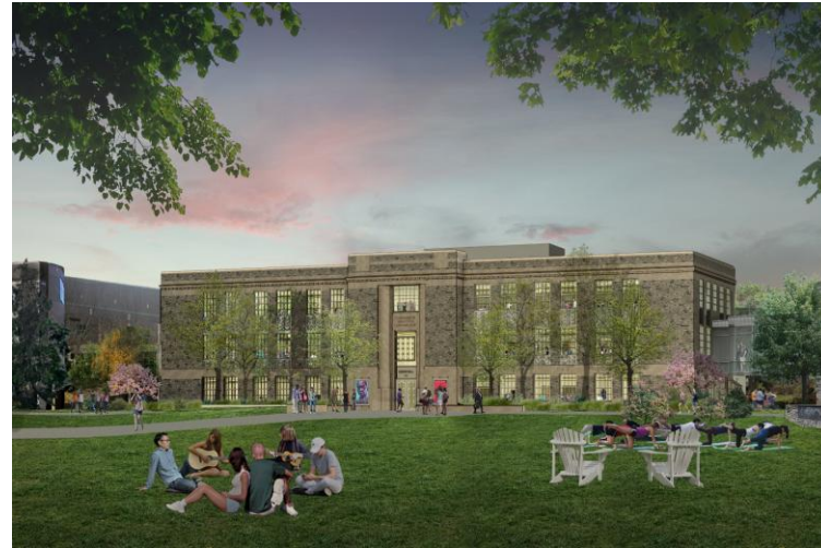
Addition/Renovation, Private Client, 1936
