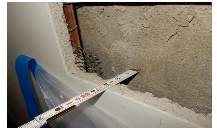
INTERIOR WALL ASSEMBLY PROBE
