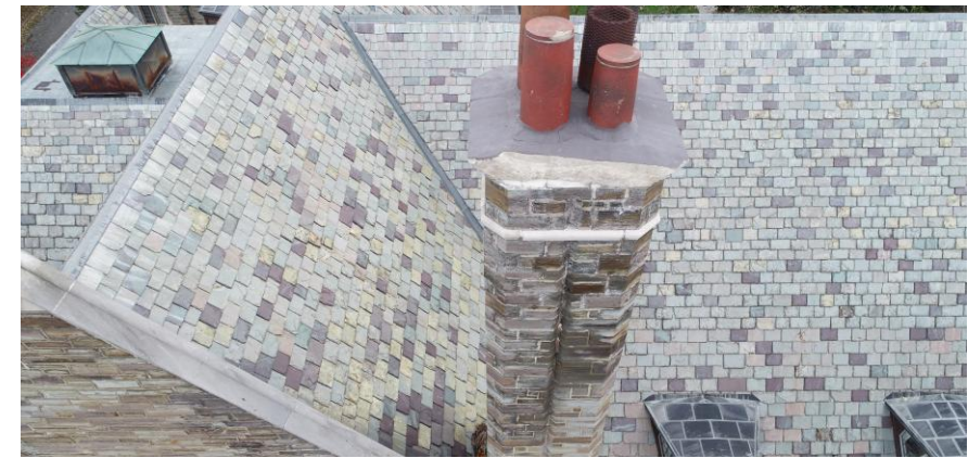
DRONE SURVEY OF ROOF
