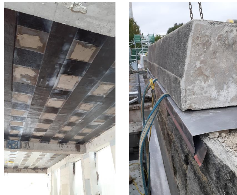
CARBON FIBER REINFORCING, PARAPET REBUILD
