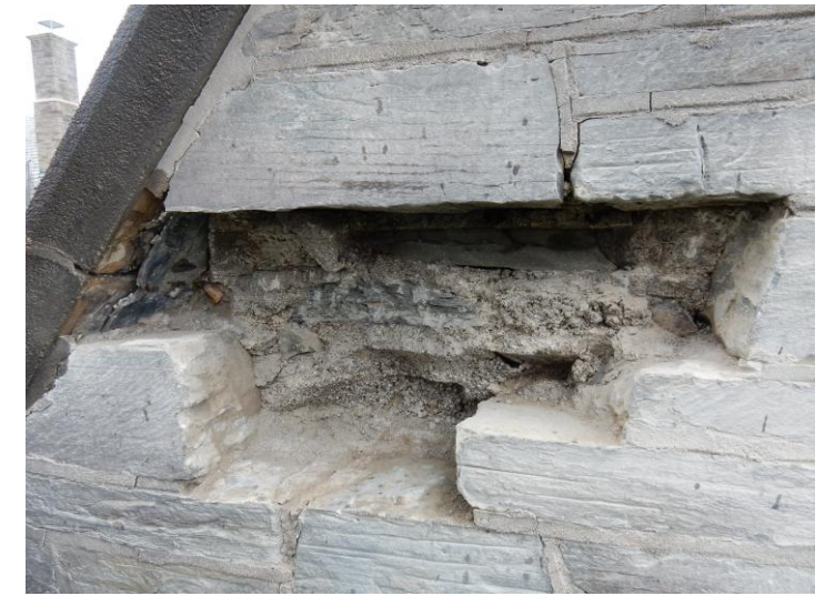
MASONRY PROBES AND SAMPLES
