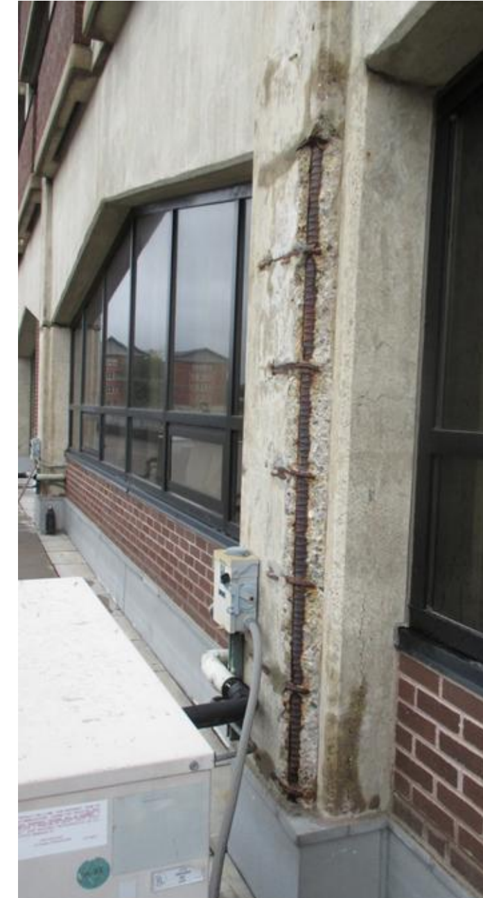
EXPOSED REBAR
