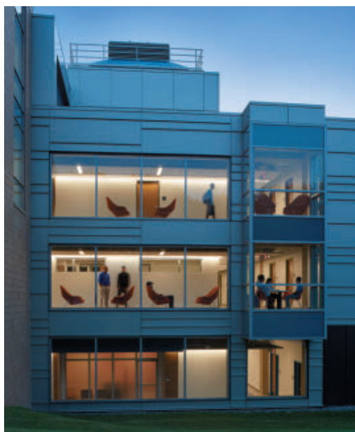
RENOVATED SCIENCE IV AT BINGHAMTON UNIVERSITY CREDIT: DAVID LAMB PHOTOGRAPHY
