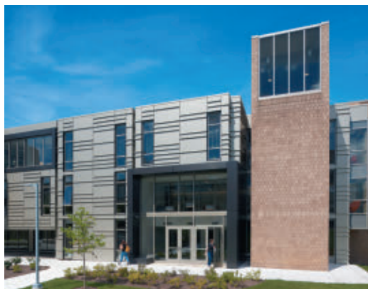
RENOVATED SCIENCE IV AT BINGHAMTON UNIVERSITY CREDIT: DAVID LAMB PHOTOGRAPHY
