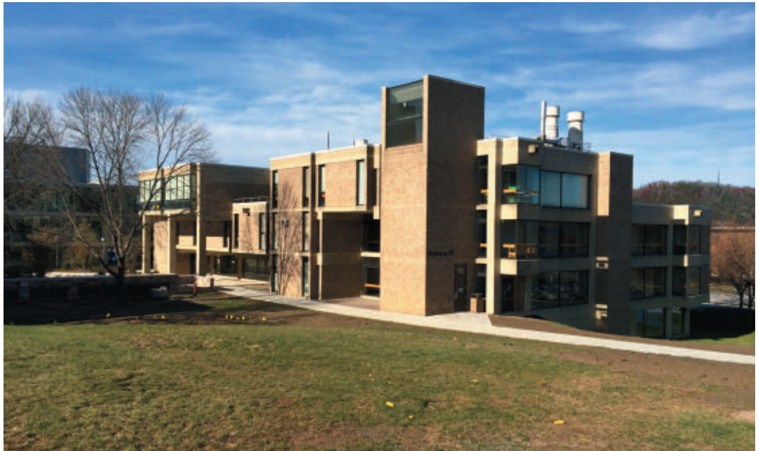
SCIENCE IV AT BINGHAMTON UNIVERSITY BEFORE RENOVATION
