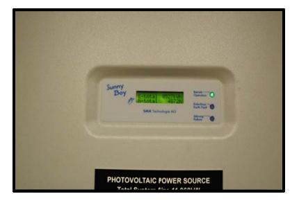
Energy Inverter for PV system 1 (Library) E-total 8,527 Kwh H-total 4,872 H
