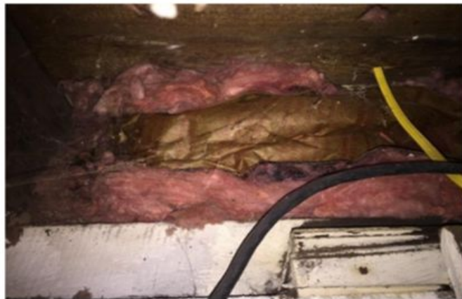
Exposed fiberglass in the basement rim joist.
