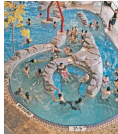
Photograph 1: If Only They Knew —Happy folks getting wet while someone else gets a financial bath. It is not easy keeping the roof and walls dry when everything else is wet.
