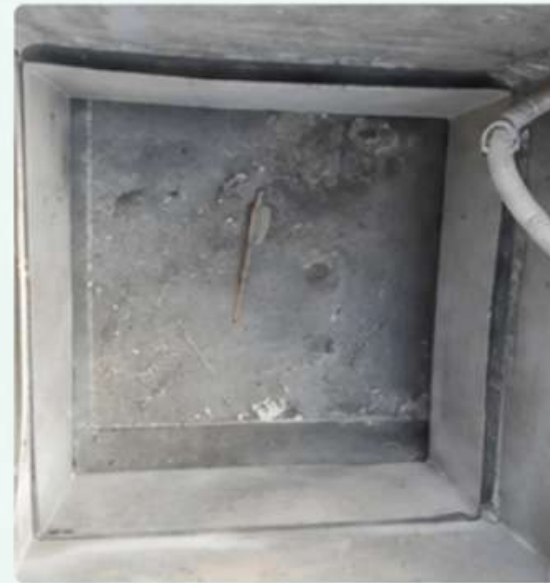
Curb Sealing (Before)
