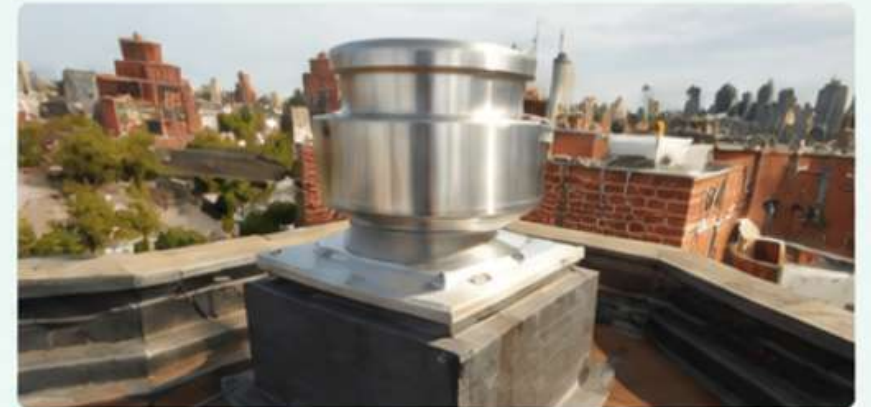
Fan Installation (After)
