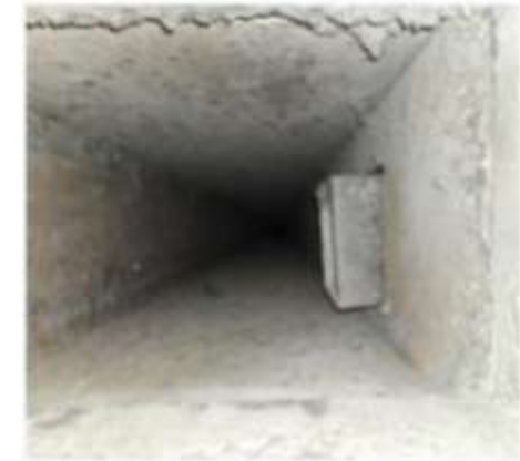
Exhaust shaft before
