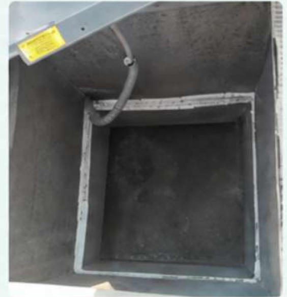
Curb Sealing (After)
