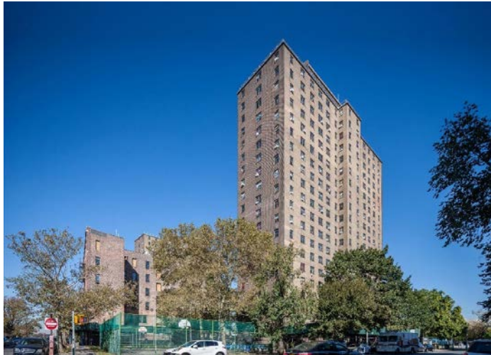
Murphy Houses - Existing
