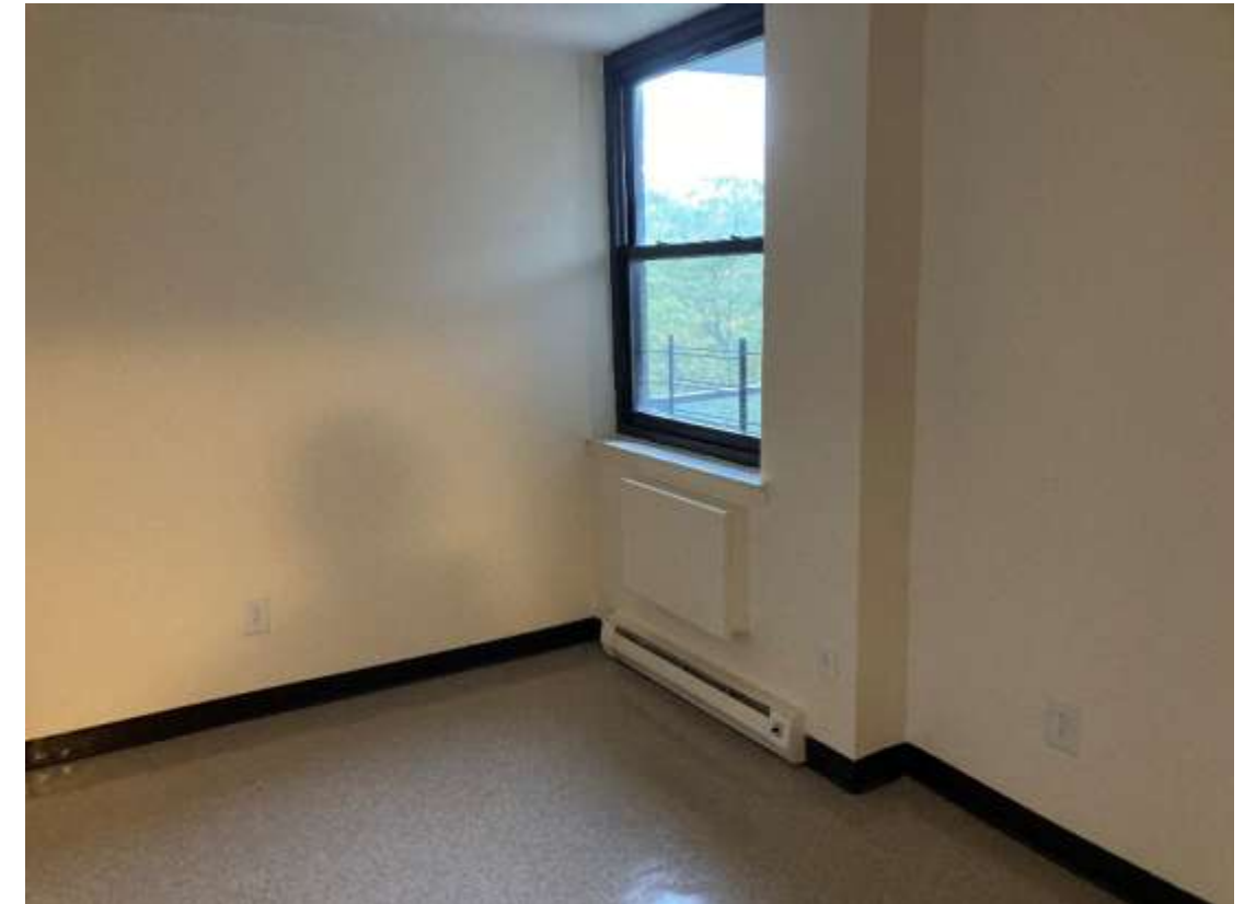
Apartment: electric baseboard below a through-wall AC sleeve
