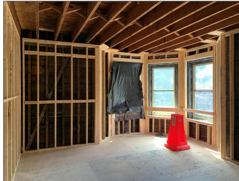
After New “Interior Wall” Framed
