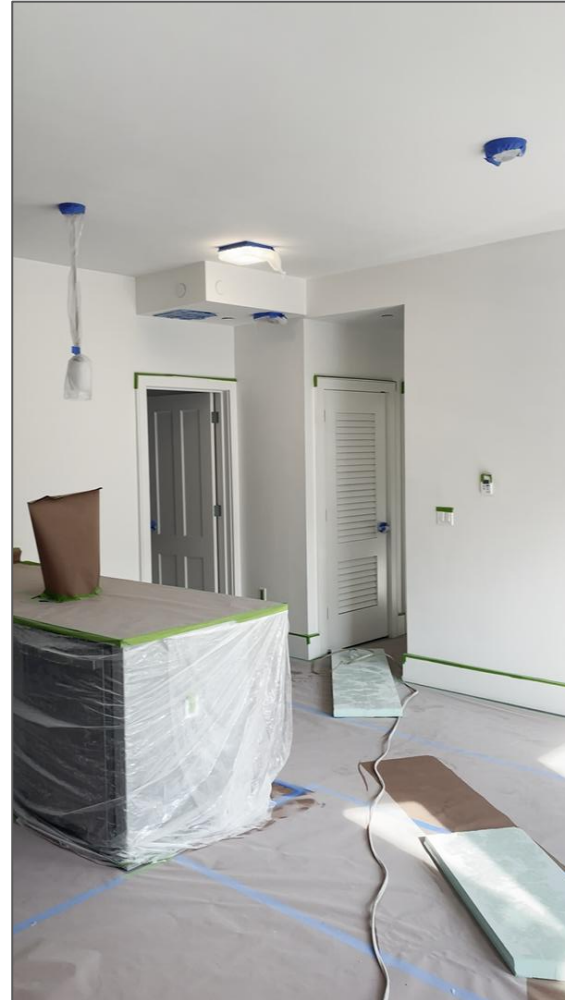
Prep Work Inside for Finished Unit
