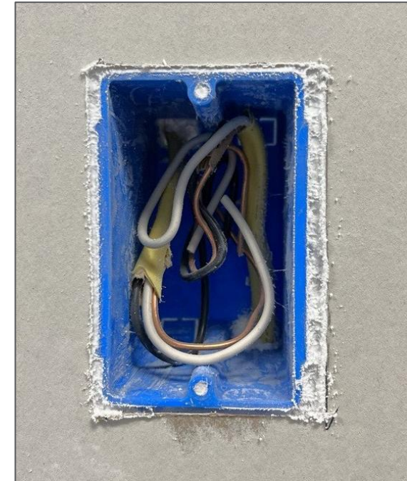
And ultimately adheres & dries only at the leakage points as a flexible sealant
