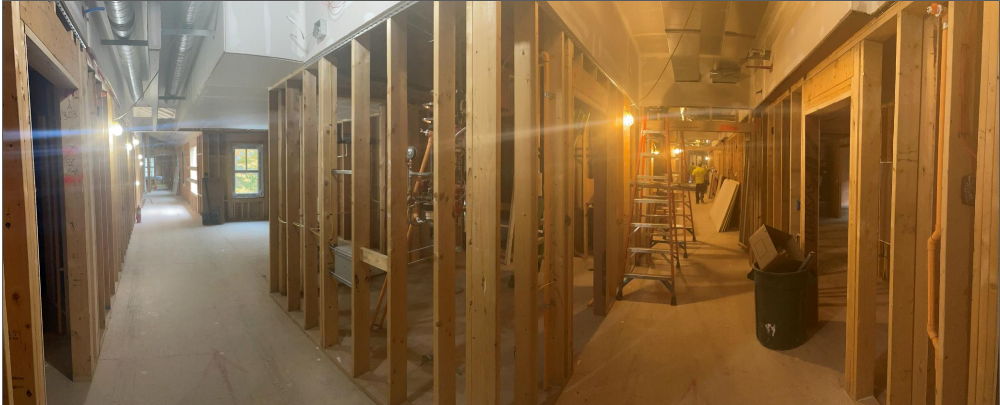
AeroBarrier seal at exterior sheathing
