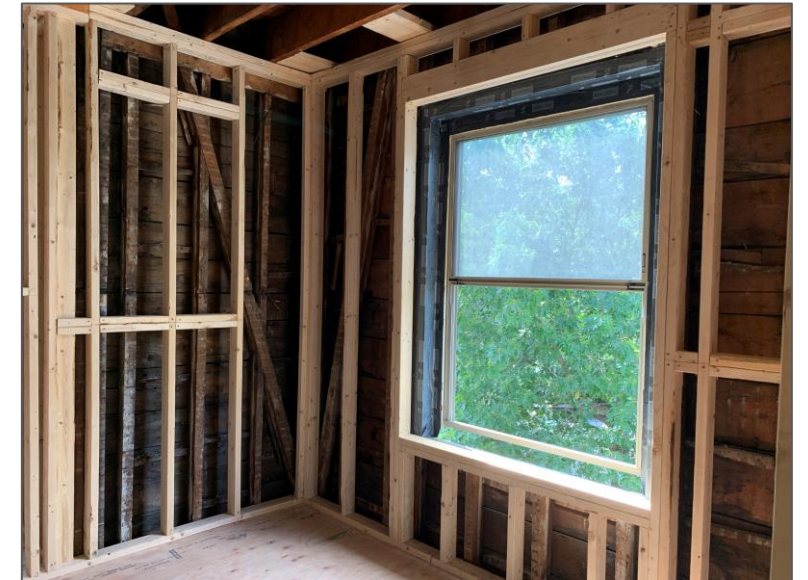
After New “Interior Wall” Framed
