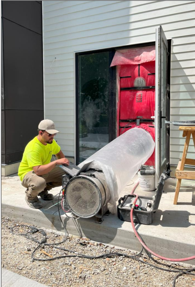
AeroBarrier Set Up Outside
