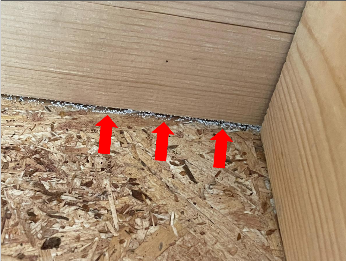
Sealant at Top Plate Exterior Wall
