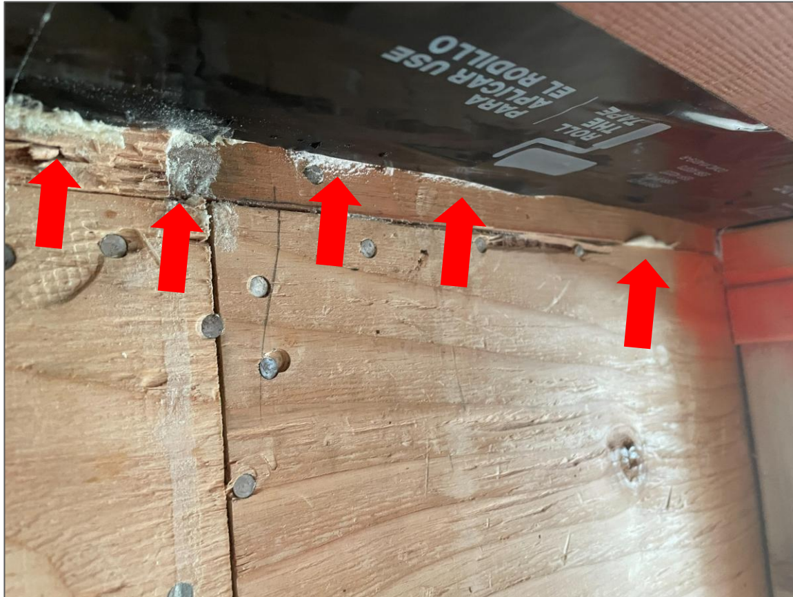
3 rd Floor Top Plate (view from side) (AeroBarrier found & sealed leakage where sealant tape installed)
