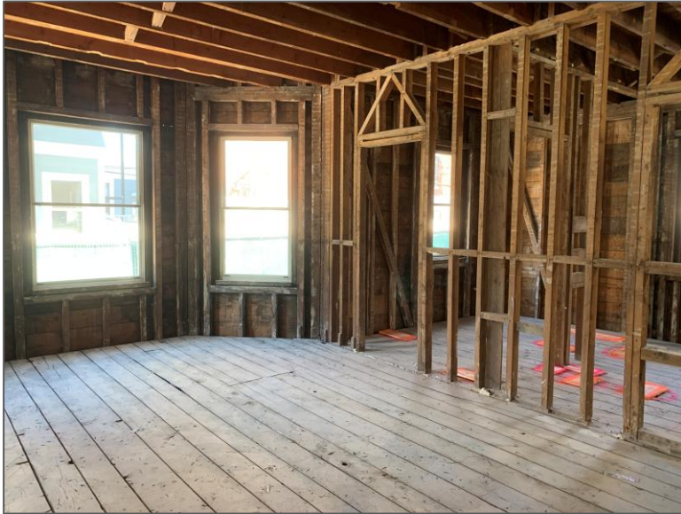
Before New “Interior Wall”
